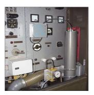
Fig. 3. Air purification filter P61 manufactured by BAUER (a); a general view of the filter installed in the air supply system of the underwater works securing base "ORTOLAN" (b), (a and b), source: (a) manufacturer's information materials, (b) own research.
